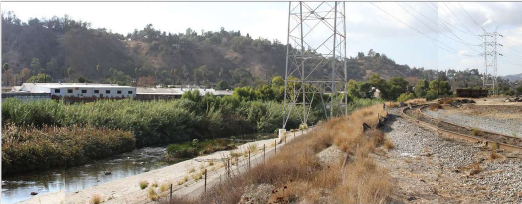
East Side- View of LA River ( Looking North)
